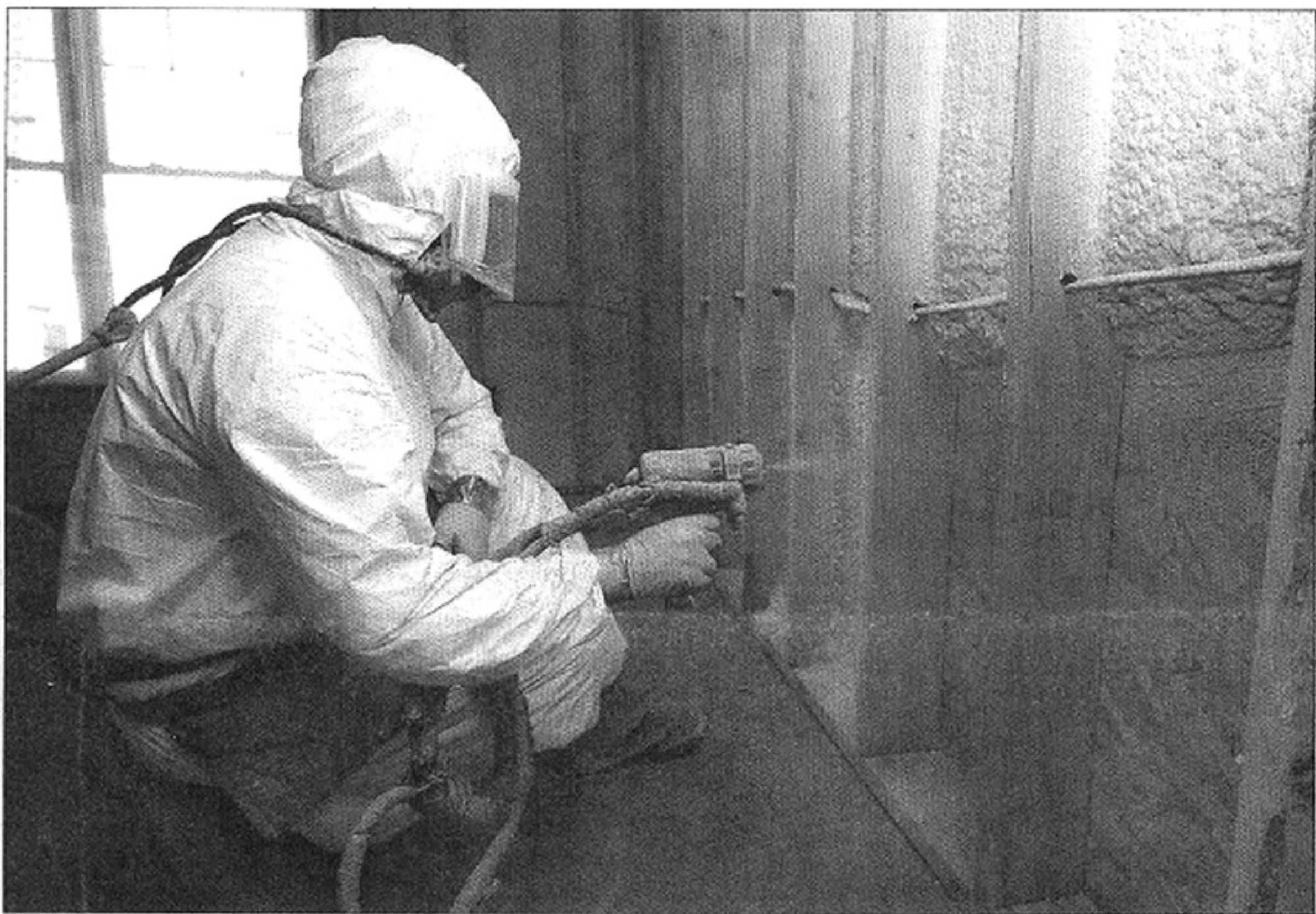
Luis Sanchez of Fairfield Insulation sprays foam insulation into the walls of a home under construction in New Milford. David W. Harple/Staff photographer
